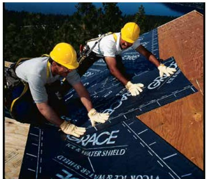
**Foldless release paper** – The foldless release paper provides multiple performance enhancements: fewer edge catches, 180° pull-back, ease of membrane cutting (single cuts) and membrane positioning, quicker “one-man installs” resulting in an easier, more productive release.
